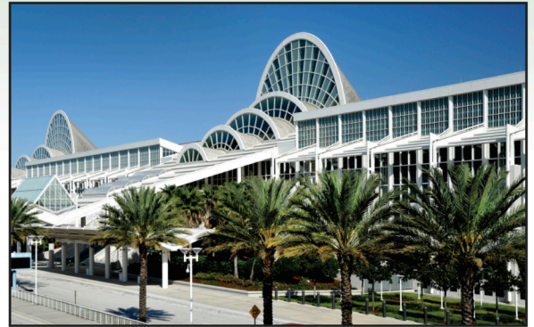
Orange County Convention Center Going Green with New Solar Panels
